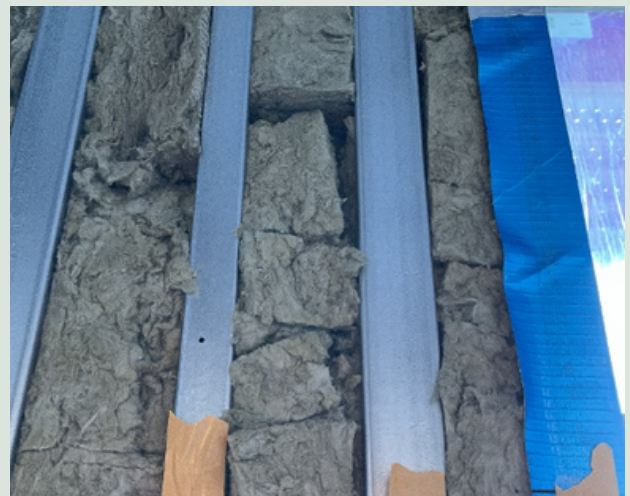
Insulation within structural zones can be tricky to maintain thermal continuity and is broken by structure and infill
