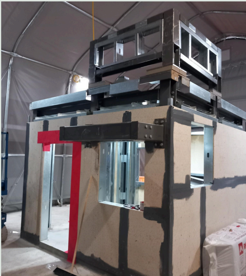
Kier Construction Test rig at Currie High School to agree best practice details and solutions with supply chain
