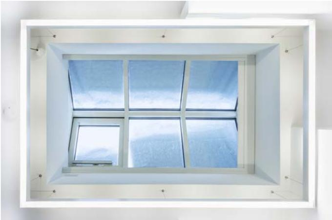
Figure 6.18 - Passivhaus certified rooflight, Feilden + Mawson LLP
