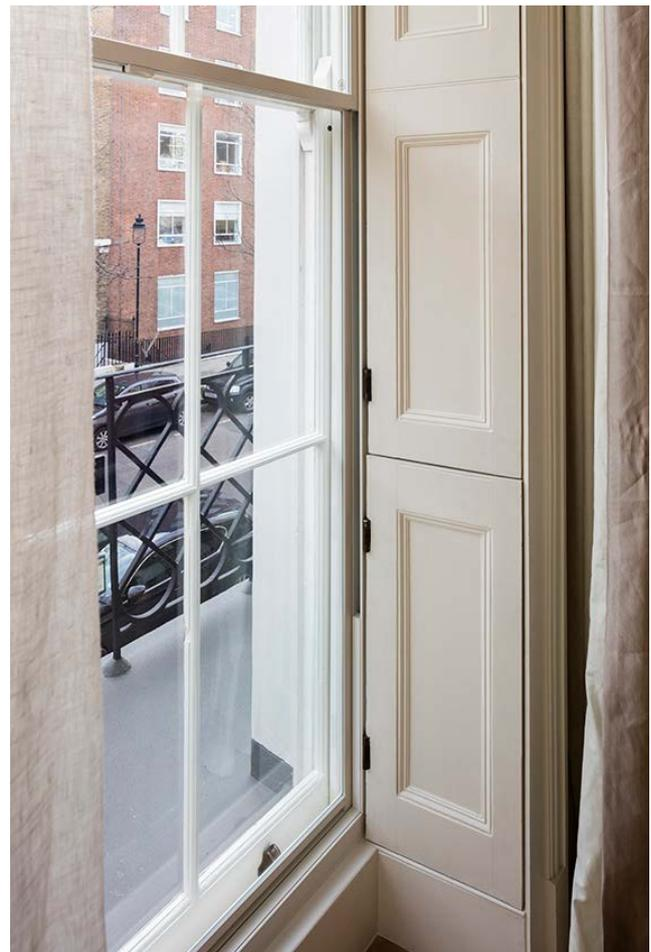
**Figure 6.29** - High performance secondary glazing post retrofit. Prewett Bizley Architects
