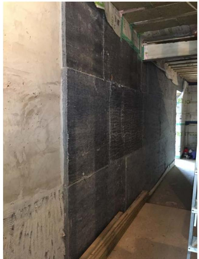
**Figure 6.20** - Installation of internal wall insulation (40mm Aerogel applied to the internal walls to minimise loss of space), Feilden + Mawson LLP
