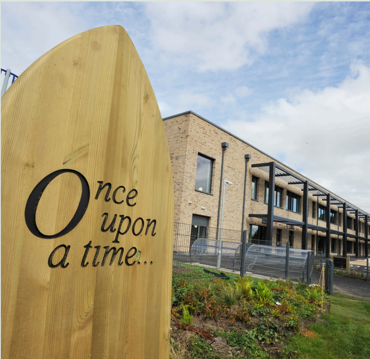
Recently completed Montgomerie Park Primary School by Robertson Construction
